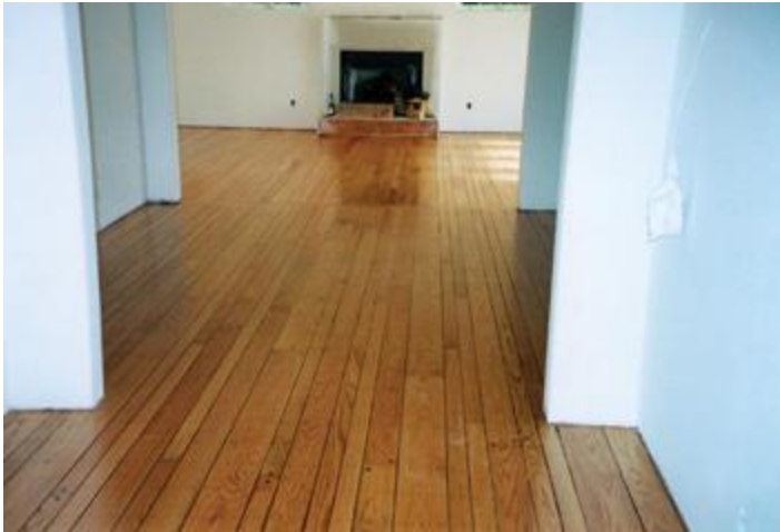
An existing top-nailed plank floor with plugs in the Bay Area.
