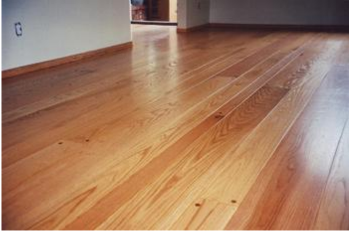
A random-width plank top-nailed wood floor with plugs.
