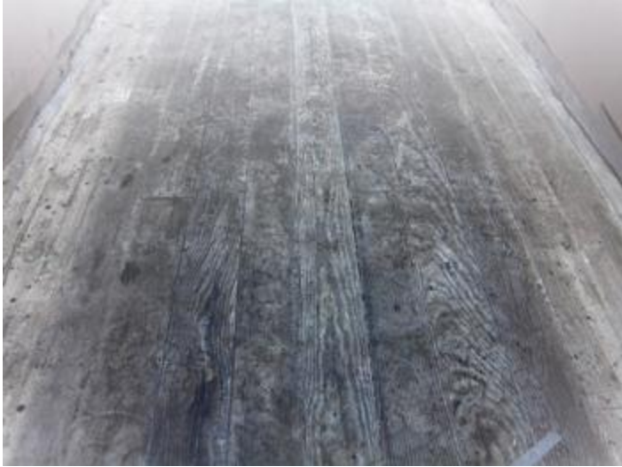
An old solid board subfloor, commonly found under 5/16-inch wood flooring.
