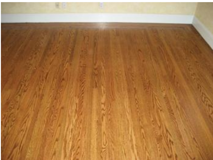
A new stained red oak top-nailed 5/16-inch wood floor in the Bay Area.
