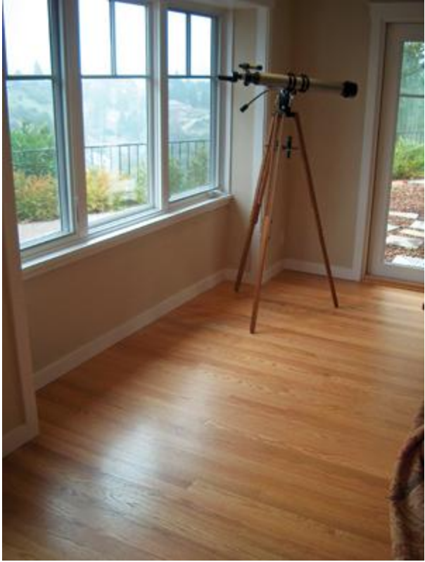
A new 5/16-inch strip top-nailed oak wood floor in the Bay Area.
