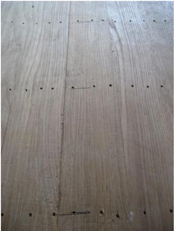
A new top-nailed 5/16-inch wood floor before sanding.
